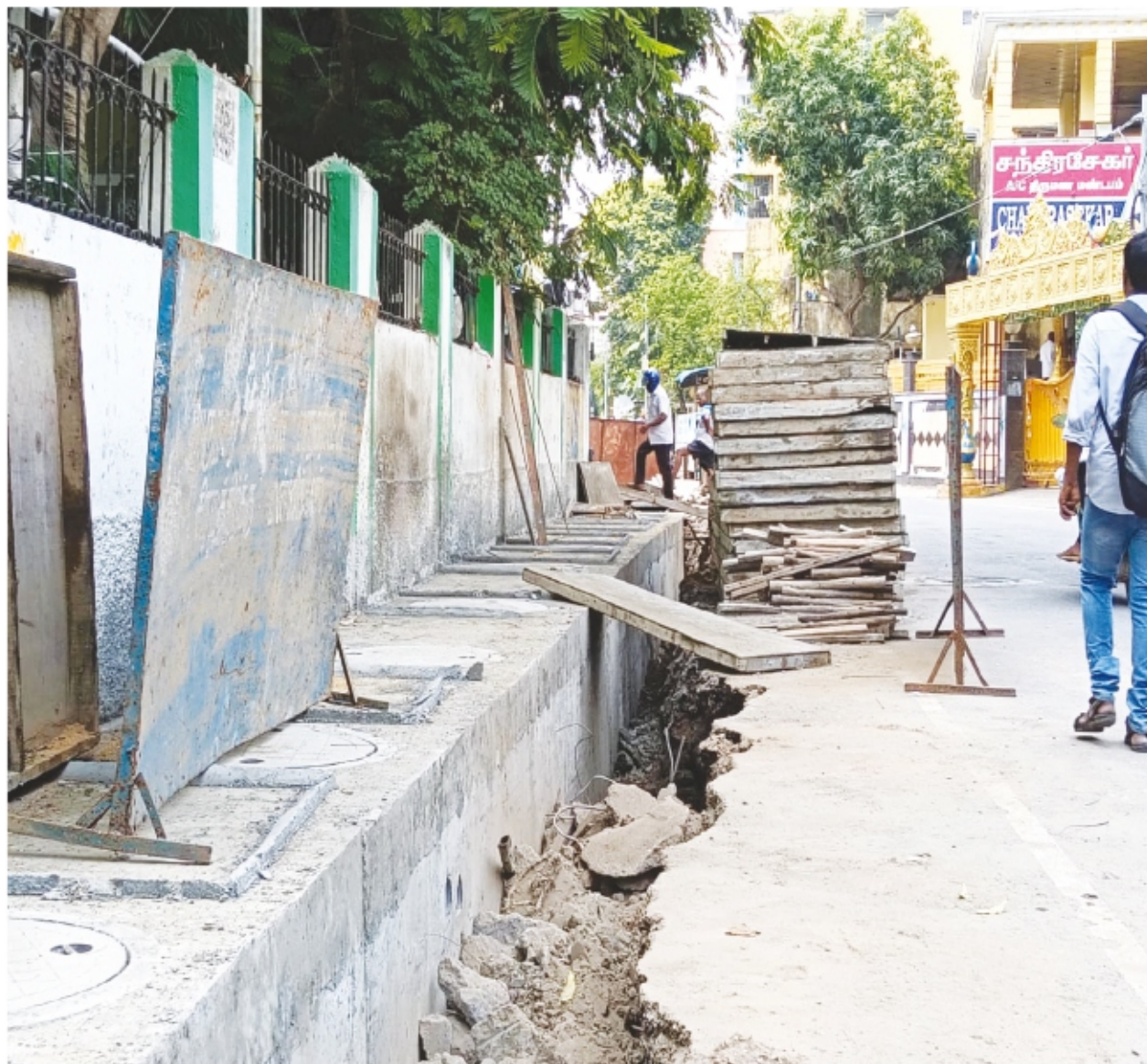
After completing the work of SWD in Kuppiyah Street, West Mambalam. The gap between SWD and the road was not covered. It will be very difficult for walkers at night time.
