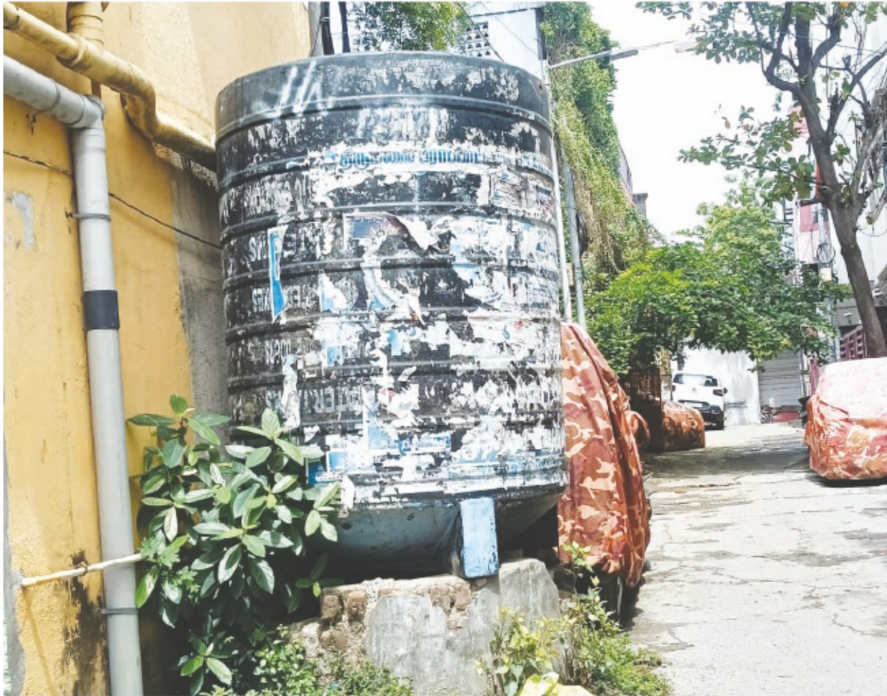
NOT IN USE : A large water tank dumped at Puspaavathi Ammal Street, West Mambalam. The tank is used only for pasting posters etc. Will the concern authorities put the tank for better use.
